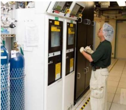
A technician collects data from two GASGUARD® cabinet AP 11 controllers, which are designed to keep the gas flowing.
